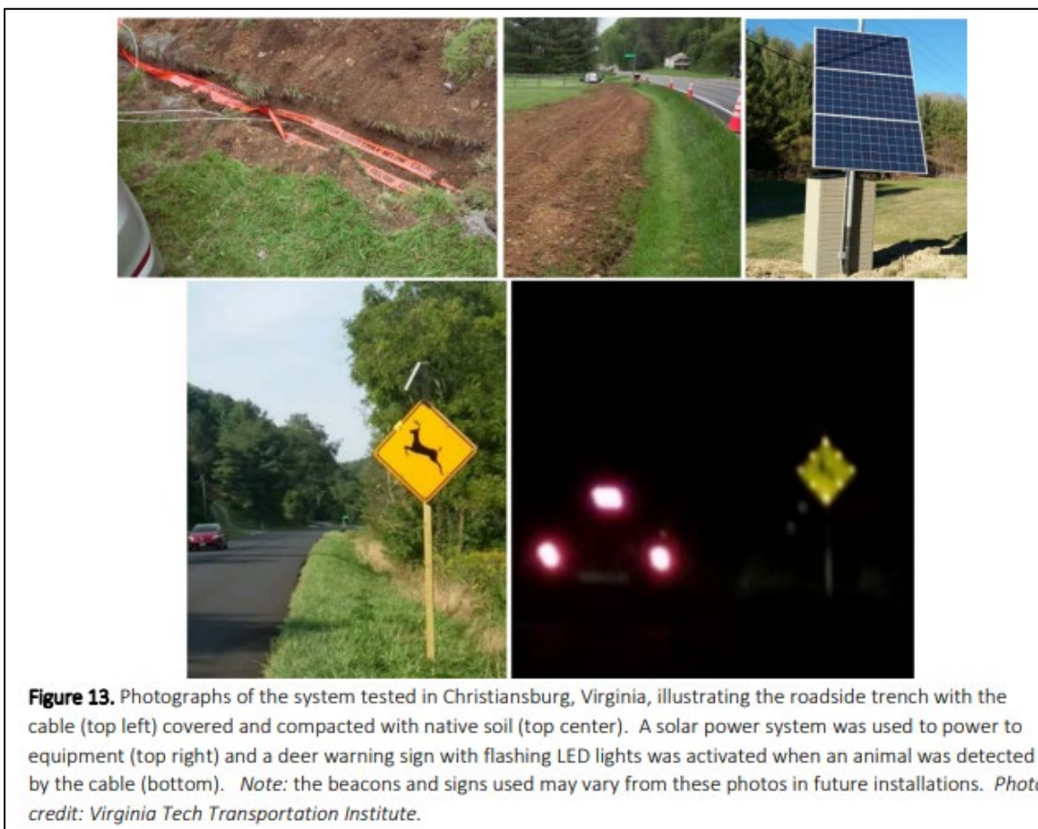
Figure 24: Animal Detection Warning System, Source: "Large Animal Crash Countermeasures in Virginia", Virginia Transportation Research Council, April 2022.
