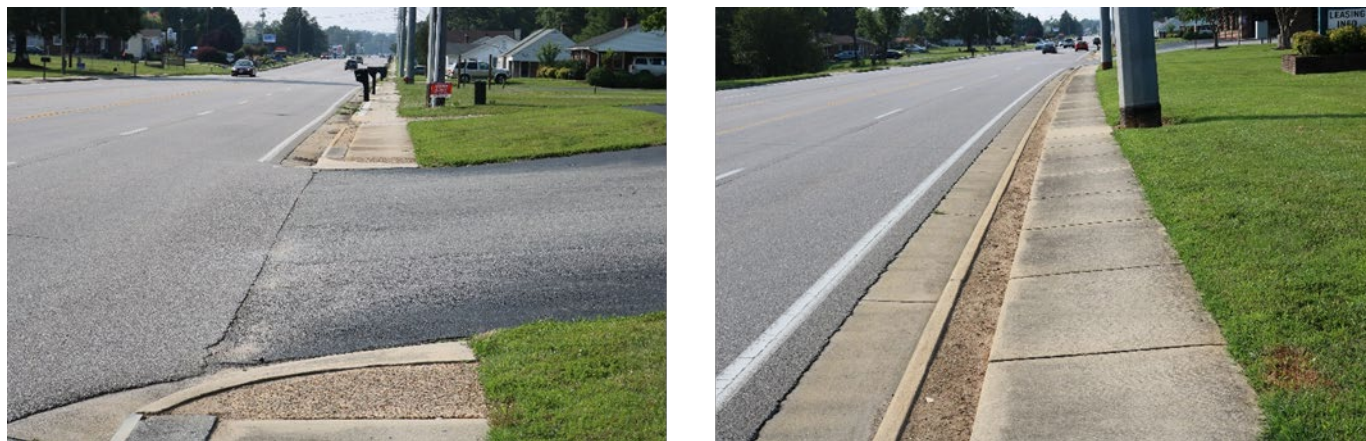
Figure 13: VA 41 Existing Sidewalks
